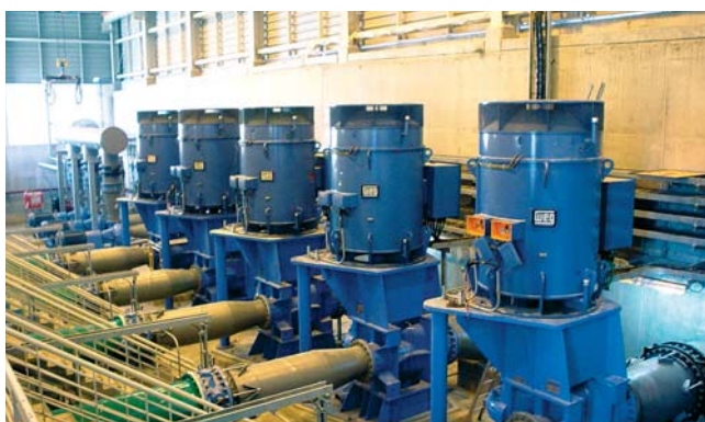
Customer: Thames Water Projects Country: Thailand
