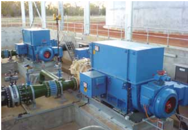
Supply: 2,000 kW, 11,000 V, 4 poles, frame 560 Application: Water pump
