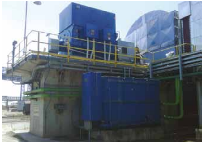
Supplies: 9,000 kW, 6,600 V, 8 poles, frame 900 Application: Exhaust fan
